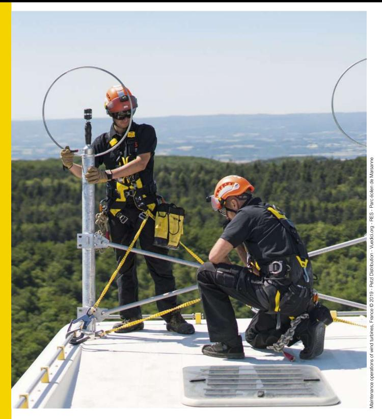
To give each user the best possible fit, Petzl harnesses are adjustable at the waist, shoulders and leg loops. They are equipped with different types of buckles:
